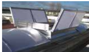
Upstand in arcade rooflight
