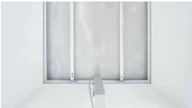
Darkening flap with M3 linear drive -view from below
