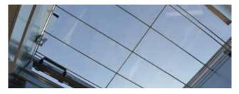
3. Kingspan Light + Air AeroTech® insulation The Kingspan Light + Air AeroTech® solution is a technology based on insulating aerogel injected into the polycarbonate walls, which improves the diffusion of natural light while reinforcing thermal and acoustic insulation.
